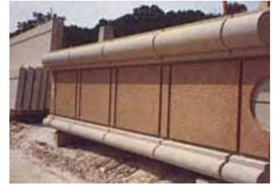
**Figure 6** Multiple mixes with sandblasted and acid-etched finishes.
