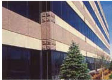
**Figure 5** Multiple mixes with acid-etched and form-liner finishes.
