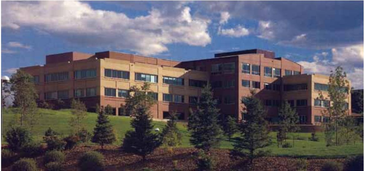
The three adjacent buildings constructed for Access Health Inc. feature precast concrete panels colored to complement the mountain backdrop and textured to resemble native Colorado red-and buff-colored sandstone shiners. OZ Architecture's design uses articulation and shadow lines to break up the mass of the panels.
