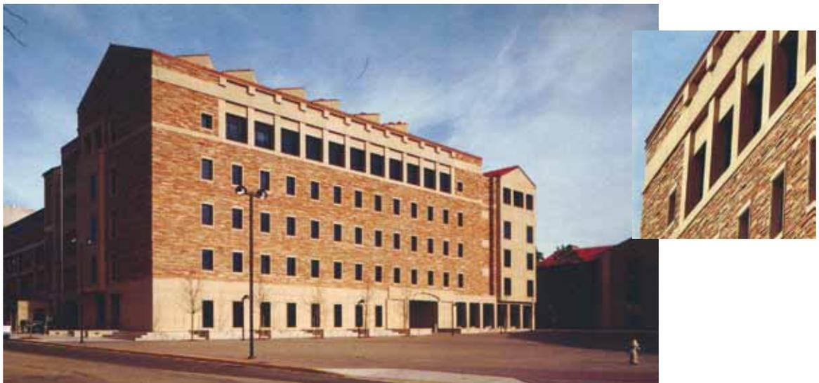
At the Molecular, Cellular and Developmental Biology (MCDB) Building at the University of Colorado in Boulder, OZ Architecture used limestone-colored, acid-etched precast base and trim to provide contrast to the campus' standard Colorado red sandstone. Stone was installed on steel studs after one-piece precast window surrounds were erected.
