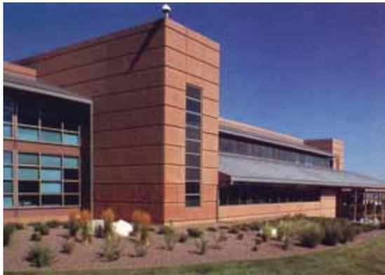
At Quantum research and development facility in Colorado, precast panels were used for their cost-efficiency and durability. The panels' articulation follows the horizontal lines of the ridge behind by using bold reveals and subtle color variations within the panels. To define the strong building base, a stone liner was used to mimic Colorado red sandstone.
