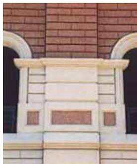
**Figure 2** Multiple mixes with retarded and sandblasted finishes.
