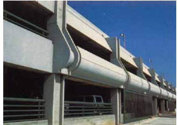
Large bullnose components added to the parking structure at the Hyperion Wastewater Treatment Facility provided a distinctive visual element that tied to the other buildings in the project without mimicking their exact look.
