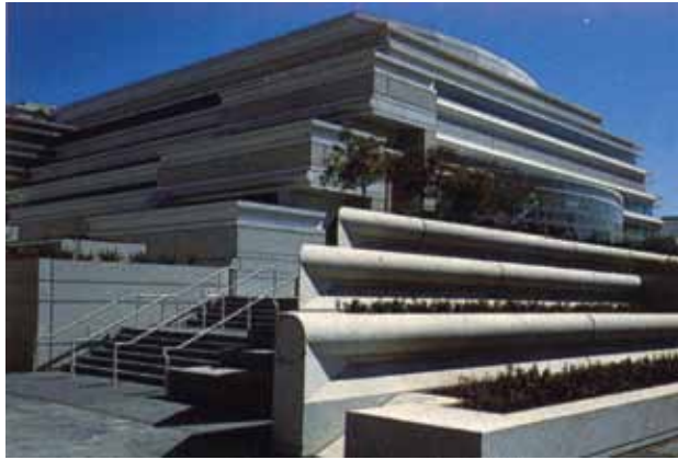
The lobby façade of the Moscone Convention Center makes ample use of bullnose sections, tying in with planters and adding visual interest to the center.
