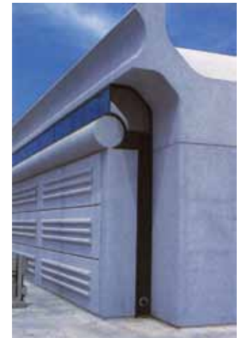
The use of the bullnose sections on various support buildings at the Hyperion Wastewater Treatment Facility broke up the flat-panel façade and created a distinctive look.
