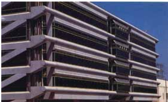
Adding bullnoses along each window ledge of the Terminal Services Building at the Hyperion Wastewater Treatment Facility added variety to the design, improved the proportions of the façade, and created changing light patterns during the day.
